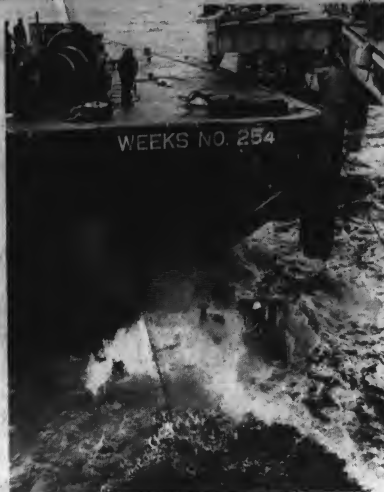
The Chesapeake Bay Bridge-Tunnel was reopened to traffic last Thursday following a two week closure after being rammed by a drifting barge. A Navy amphibious bulldozer pushed the barge away from the damaged bridge, after efforts to refloat it failed, to allow repairs to the damaged span to begin. (Navy photo by PH1 Bill Pointer)
